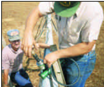
Figure 13. Installing swedge coupler.
