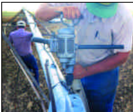
Figure 12. Drilling for swedge coupler.
